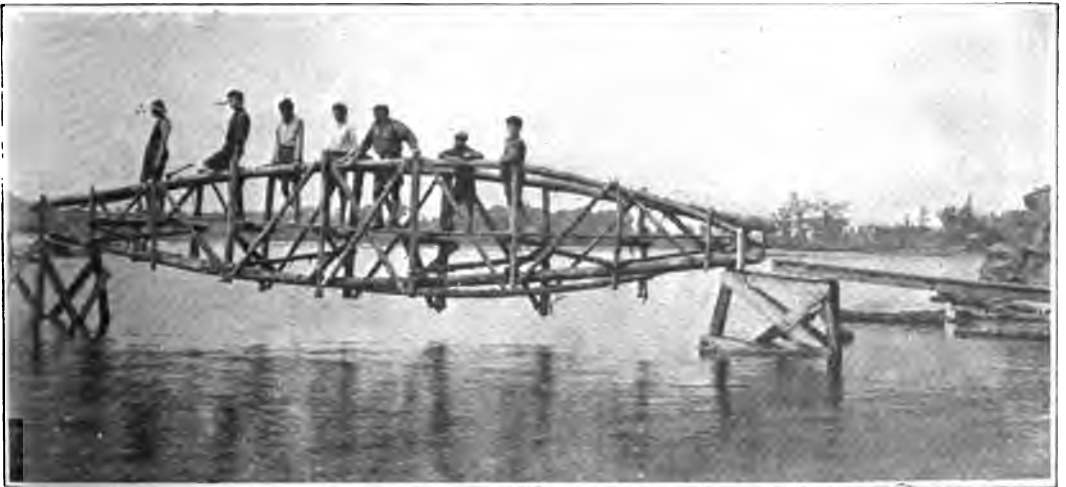
SECOND BOWSTRING SPAN IN POSITION, SHOWING PIERS ON WHICH IT RESTS
